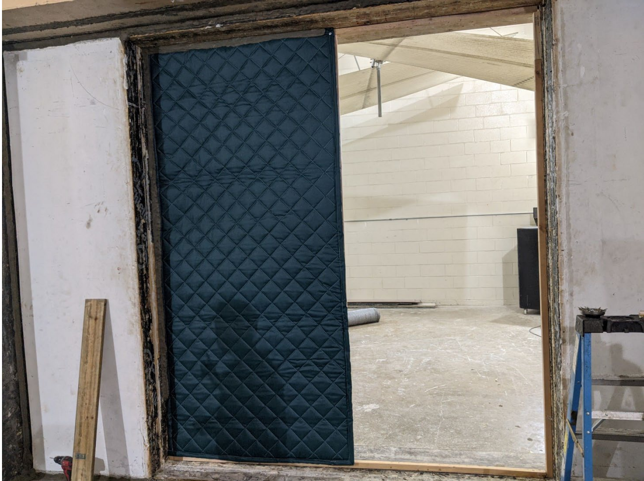
Figure 3 – Individual specimen blanket prior to perimeter sealing
